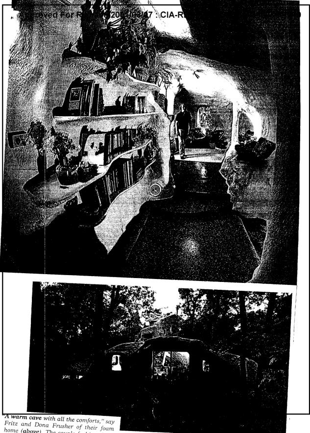
structure by inflating plastic sheets and spraying them, 6 to 8 inches thick, with polyurethane, a material used as insulation. A small forced-air furnace heats the house at a fraction of the cost for a conventional dwelling. The free-form structure seems to melt into its environment of their force.
