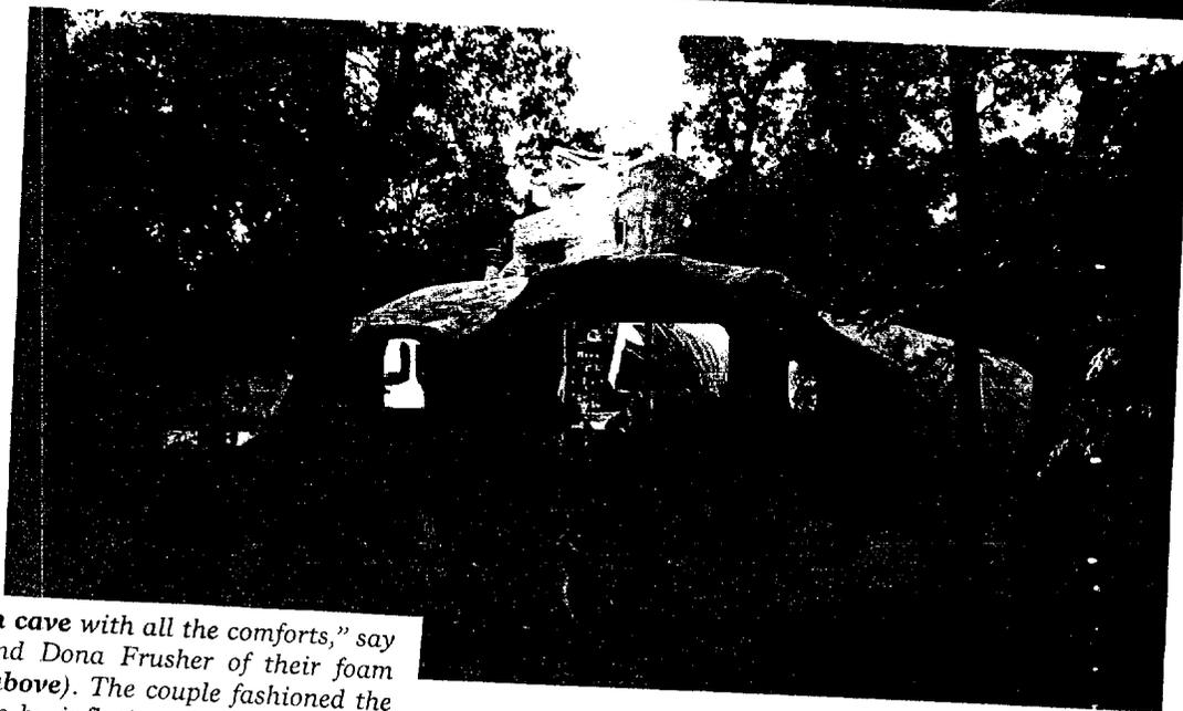
*"A warm cave with all the comforts," say Fritz and Dona Frusher of their foam home (above). The couple fashioned the structure by inflating plastic sheets and spraying them, 6 to 8 inches thick, with polyurethane, a material used as insulation. A small forced-air furnace heats the house at a fraction of the cost for a conventional one. The free-form structure seems to melt into its environment, a rocky*
