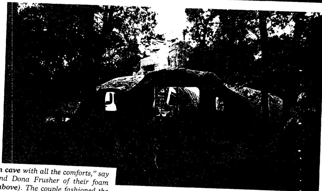
*"A warm cave with all the comforts," say Fritz and Dona Frusher of their foam home (above). The couple fashioned the structure by inflating plastic sheets and spraying them, 6 to 8 inches thick, with polyurethane, a material used as insulation. A small forced-air furnace heats the house at a fraction of the cost for a conventional home. The free-form structure seems to melt into its environment, a rocky*
